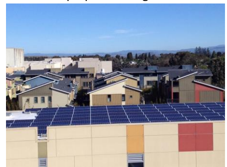
East-facing view of rooftop panels
