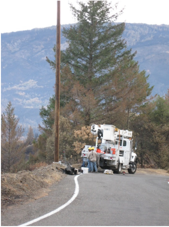
Palo Alto Utility Workers Help Rebuild 21kv line
