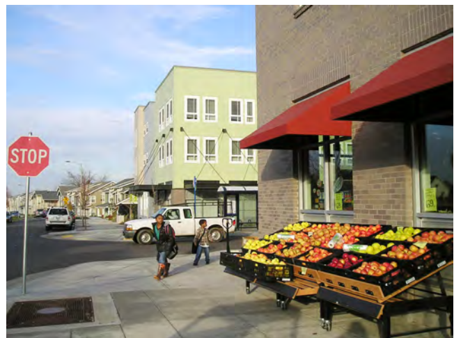
Homes in Portland, Oregon's New Columbia neighborhood are close to amenities such as a grocery store, parks, the Rosa Parks Elementary School, community college classrooms, and a Boys and Girls Club. Photo courtesy of Housing Authority of Portland.
