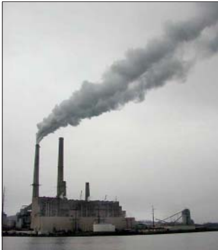
Virginia Electric Power Company's coal-fired plant at Mt. Storm, West Virginia. Source: State of New York Web site.
