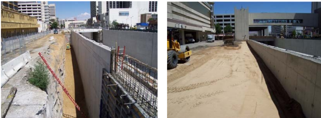
Figure 43 A second example of an operation measured as a visual percent complete. The image on the left is the current state and the image on the right is the finished state. What is the current percent complete, 25%? Is the table illusion similar to this view, Figure 66 page 356? What if the field engineer measures completion from different vantages for each location and iteration?
