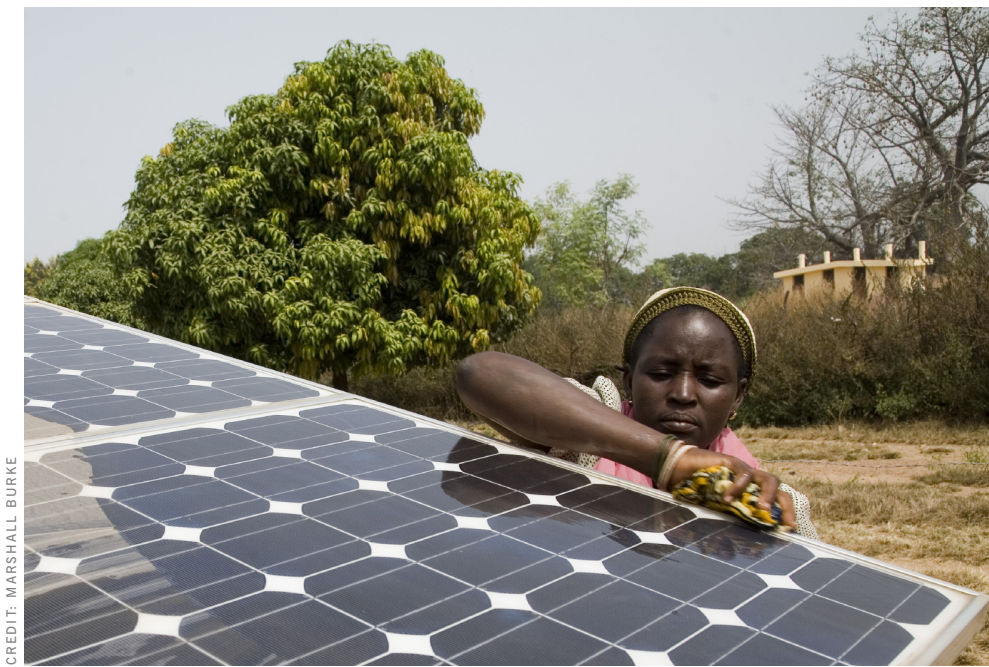
PROJECT TECHNICIAN CLEANING SOLAR-PANELS FOR SOLAR-POWERED MARKET GARDENS, BENIN
