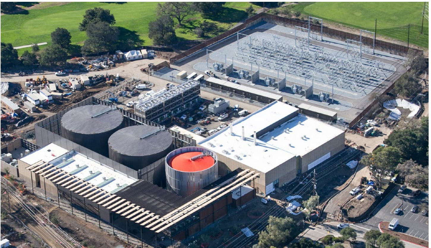
Photo: SESI represents a transformation of university energy supply from 100 percent fossil-fuel-based combined heat and power plant to grid-sourced electricity and a more efficient electric heat recovery system
