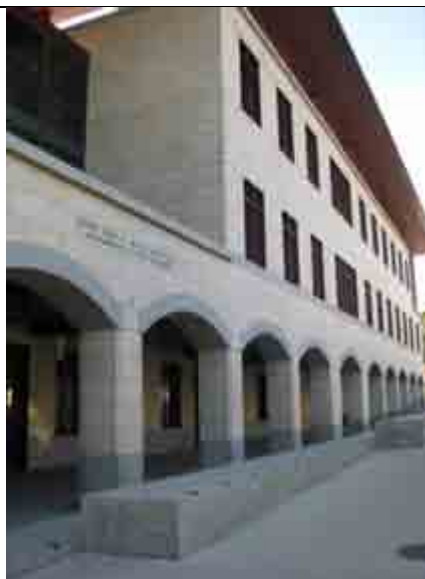
Y2E2 west side entrance
