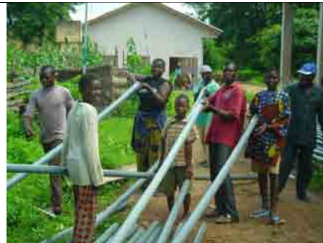
Villagers assist with the building of solar panel.
