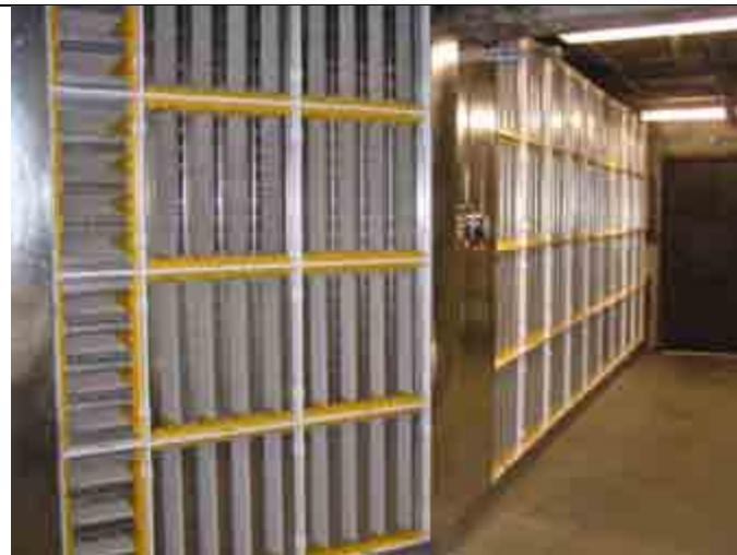
Durand Filter Racks Replacement
