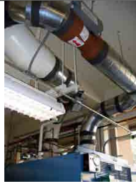
Example of the new phoenix valve (1 for each fume hood), which now allows variable air flow into the lab space
