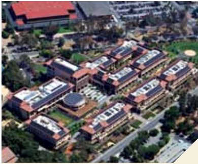
The Knight Management Center, home to the Graduate School of Business, is designated LEED Platinum for New Construction.
