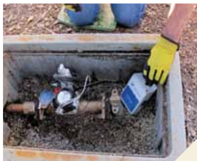
New real-time monitoring technology has helped stem water leaks, resulting in a 38% decrease in irrigation leaks.
