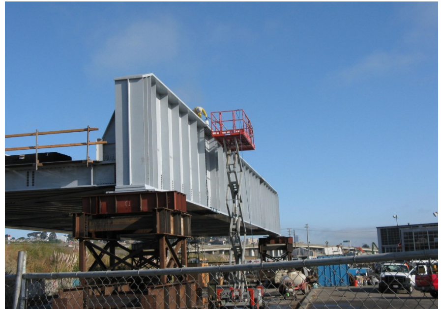
Jerrold Street Bridge - 2011
