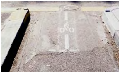
Figure C-2: Bicycle-sensitive loop detector
