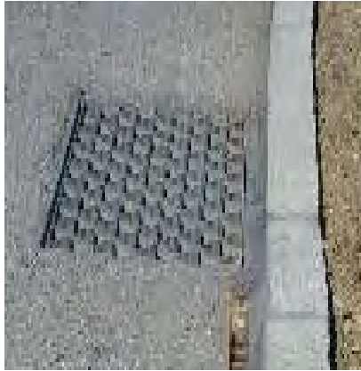
Figure C-1: Bicycle-safe drainage grate
