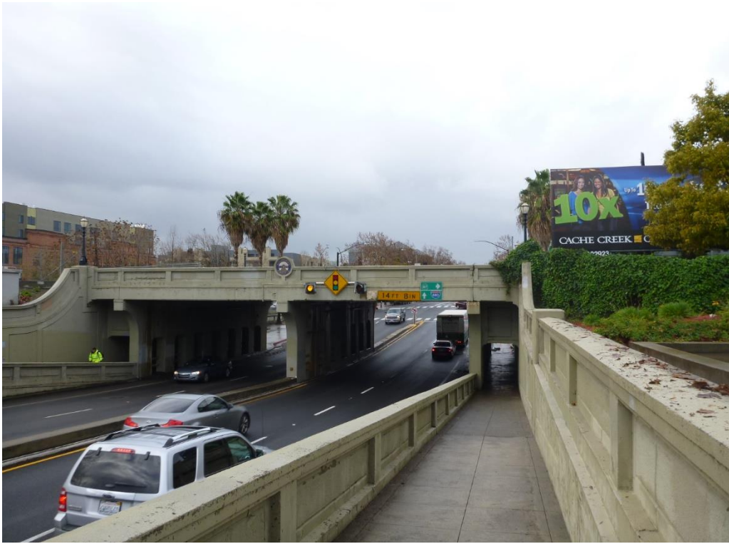
Photo 3: Santa Clara Street bridge crossing, facing west.
