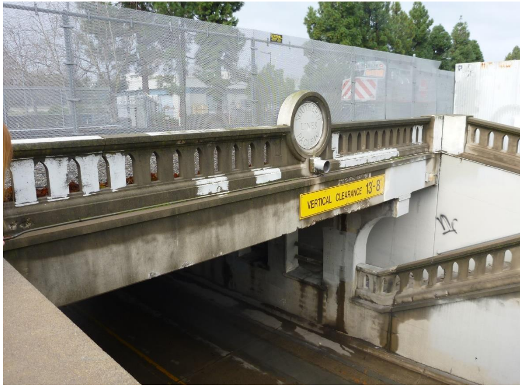
Photo 5: Julien Street bridge crossing, facing northwest.
