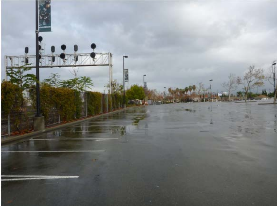
Figure 6: View of the project area within the SAP Center parking lot (note existing signal bridge on left)
