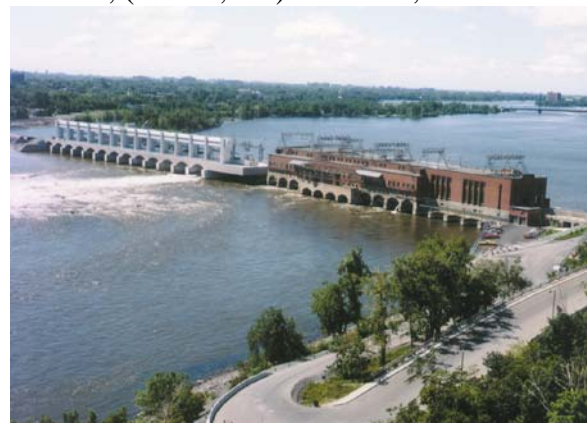
Low head power plant (45MW) Rivières-des-Prairies, (head 7,5 m) Montreal, Canada
