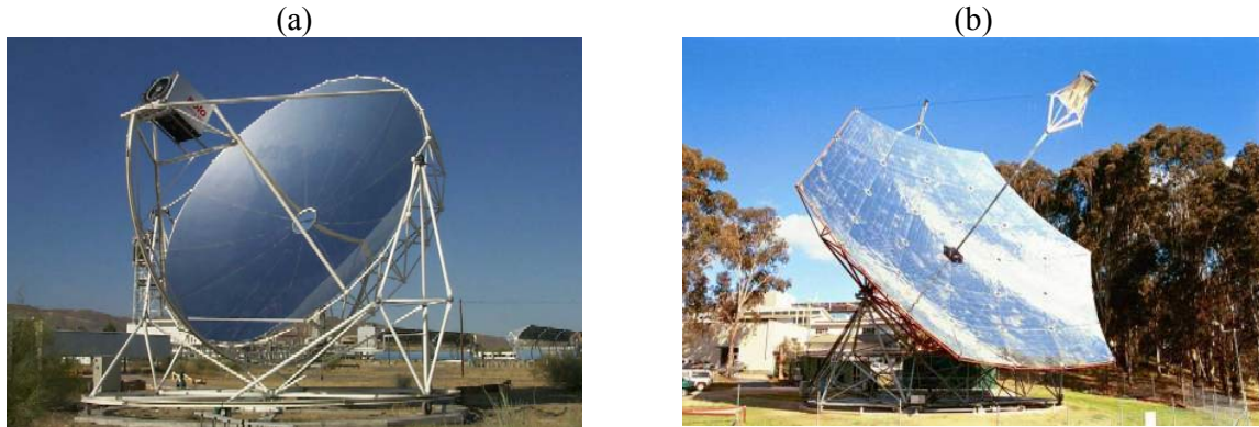
2 Figure 3.15: (a) Photo of a typical dish/Stirling system, and (b) a 400-m 2 dish system at Australian 3 National University in Australia.
