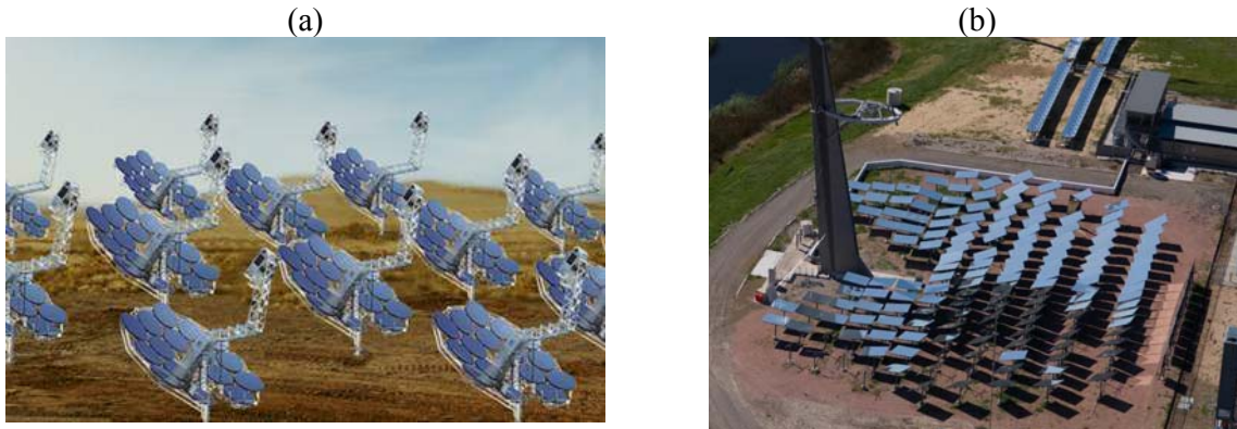
6 Figure 3.16: (a) Rendering of aggregated dish/Stirling units, and (b) a sister tower of one to be 7 used for powering a Brayton cycle microturbine (courtesy CSIRO).
