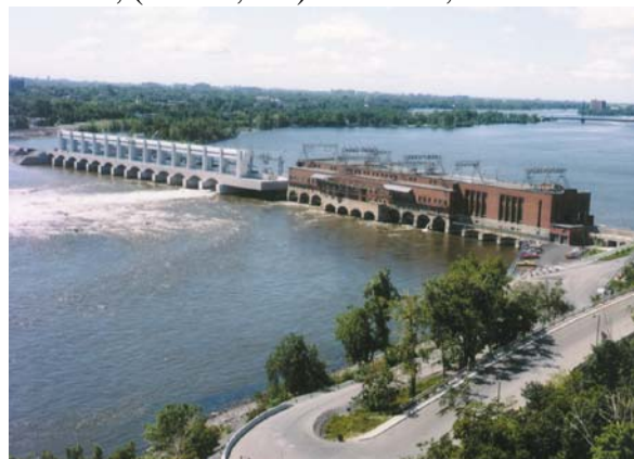
Low head power plant (45MW) Rivières-des-Prairies, (head 7,5 m) Montreal, Canada
