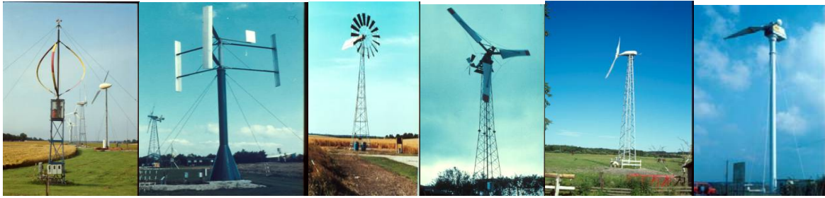
Figure 7.4. Early wind turbine designs.
