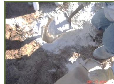
Pouring dry CZ in borehole
