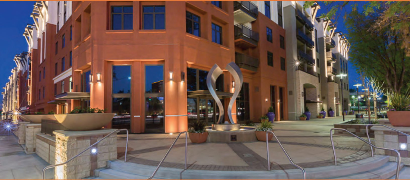
A dramatic view of Nineteen800, a mixed-use development
