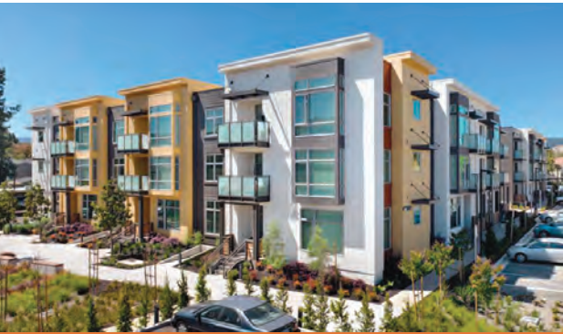
Nearing completion – Biltmore Adjacency Mixed-Use Development
