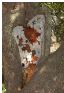
Filled tree cavity Photo: University of Florida
