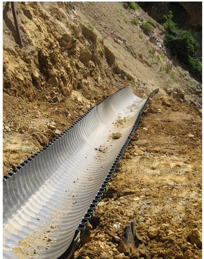
2008 – Installation of permanent portal discharge diversion structure
