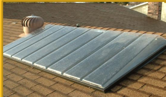
Polymer Solar Water Heaters
