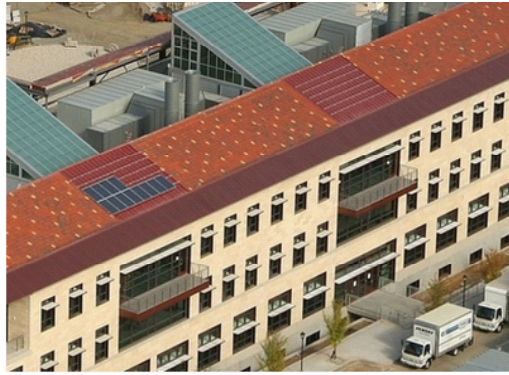
The solar panels are mounted along the south facing roof
