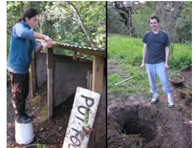
Students working on Synergy's water catchment system
