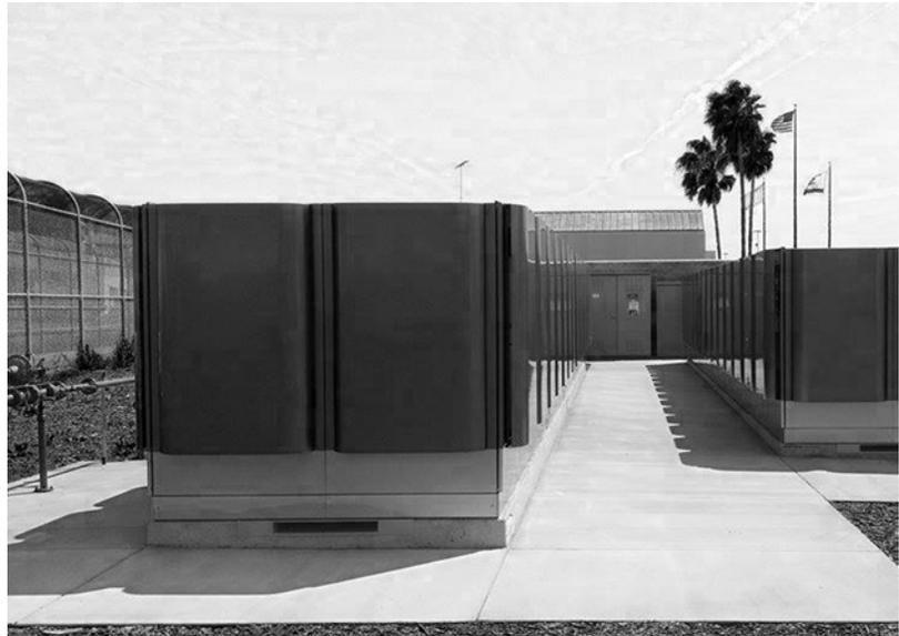
The Fuel Cell system installed at the Elmwood Correctional Facility is an 800 kilowatt system that generates 7 million kilowatt-hours of clean electricity each year, while saving the County an estimated \$2.5 million over the 20 year Power Purchase Agreement under which it was installed.
