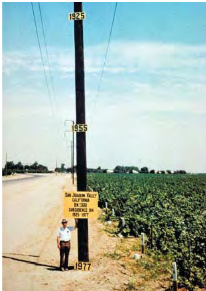
Illustration of subsidence in the San Joaquin Valley of California. (Source: U.S. Geological Survey, 1977)
