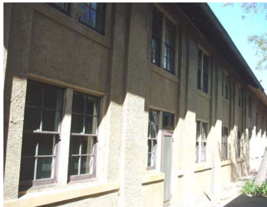
6- South Façade (western side), 2005
