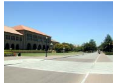
Serra Mall at Main Quad, 1999 (Sebastian & Associates)
