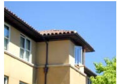
Kimball Hall roof overhang, 1991 (BAR)
