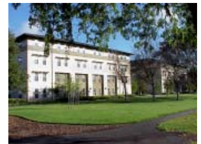
EV Infill Units, 2001 (Solomon Architecture/James Guthrie & Associates)
