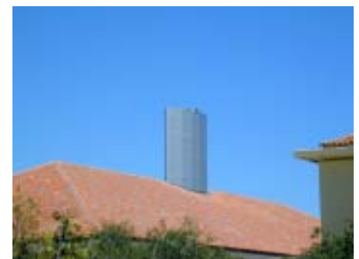
Moore Building roof stack, 2000 (Pei Cobb Freed and Partners)
