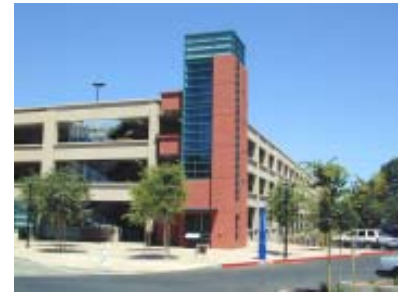
Parking Structure V, 2002 (ELS Architects/Peter Walker and Partners)
