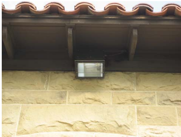
Memorial Court Arcade Eave, Main Quad
