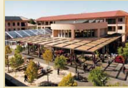
The Knight Management Center, new home to the GSB, has 4,643 on-site solar PV modules, producing 12.5% of the facility's energy.
