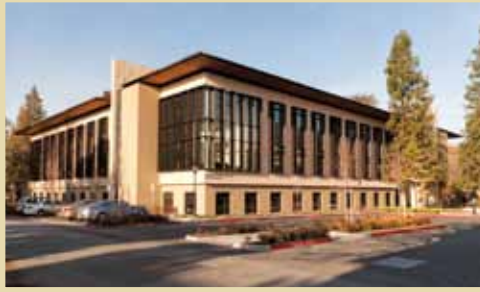
The William H. Neukom Building at the Stanford Law School is projected to use 30% less energy than required by code.
