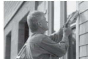
Property owner keeping his property in good repair.
