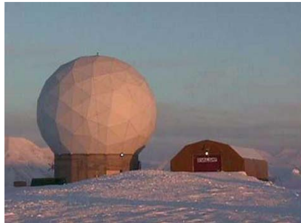
Svalbard Ground Station, Longyearbyen, Spitzbergen, Norway
