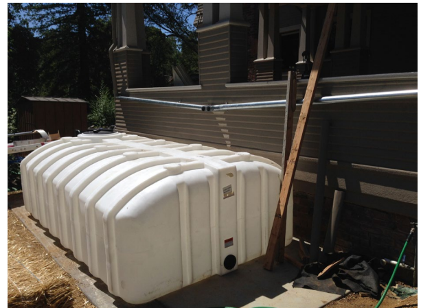
Above- This 1500 gallon rainwater catchment tank will reduce potable water usage at at Synergy House
