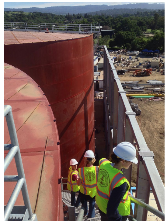
Above- GSB Students touring the new Stanford Energy Systems Innovations (SESI) Central Plant
