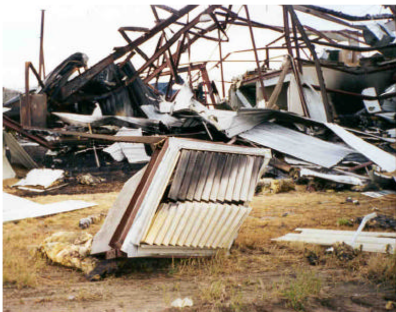
Figure 8. Ventilation Fan with Yellow Residue
