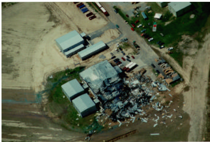
Figure 6. Aerial Photo BPS Unit Two
