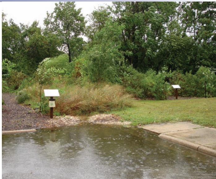
Rain gardens capture rainwater, thereby reducing stormwater runoff and conserving natural resources.
