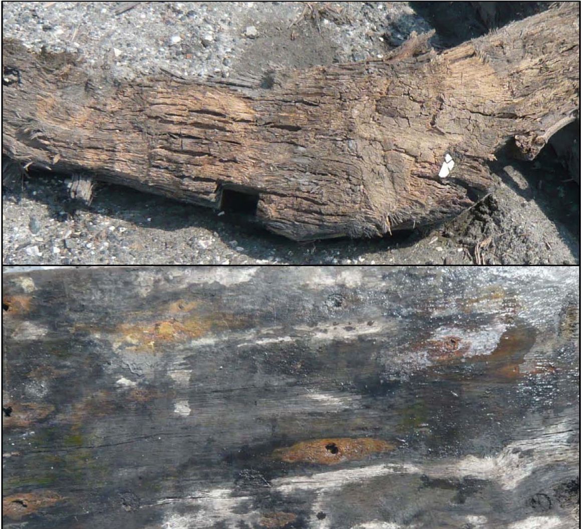
Figure 1-13. Recovered ship timbers inspected on July 16, 2009 were in generally poor condition, their surfaces split and checked from shrinkage caused by their exposure to air (top image). Preservation of the ship's iron fasteners, even in the timbers recovered in November 2009 that were kept wet prior to their documentation, was minimal with holes and rust stains providing the primary archaeological evidence of their existence (bottom image) (photographs by David Robinson).
