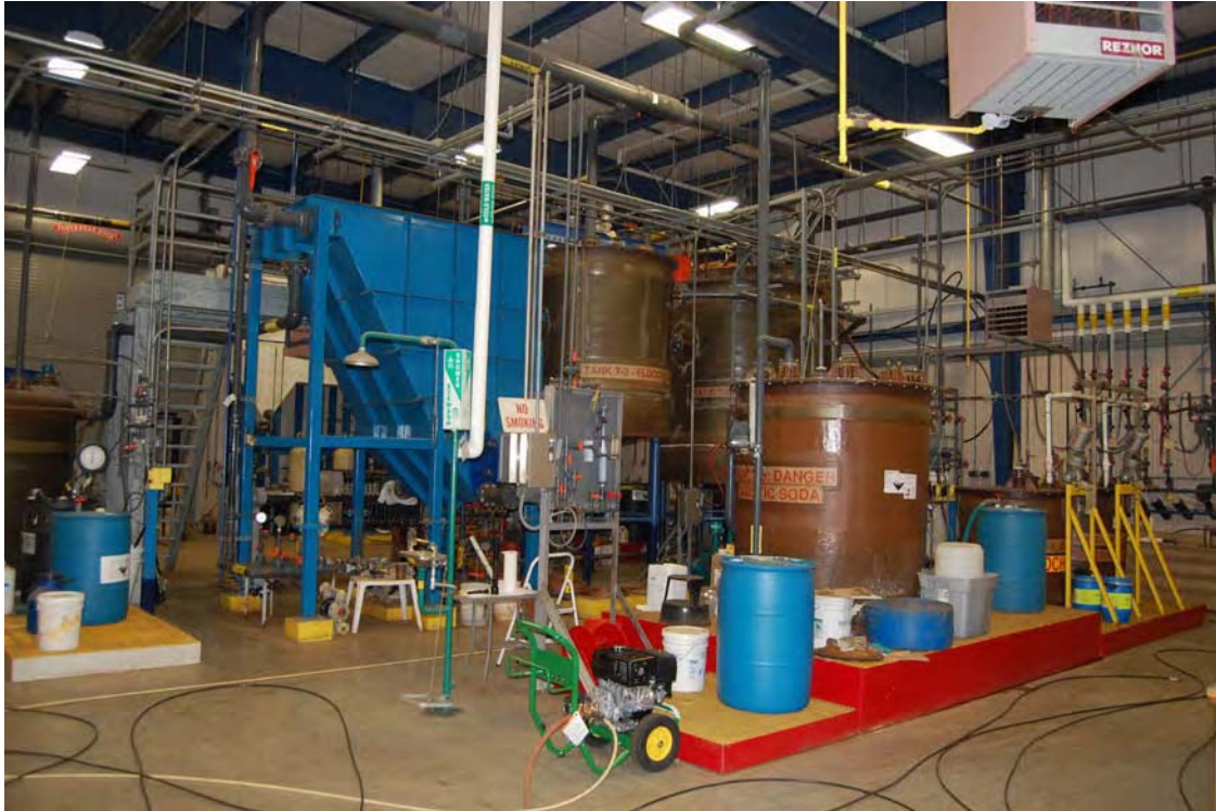
Photo Number: 10 - Air-stripper, multi-media filters, backwash tank. Date: May 29, 2008
