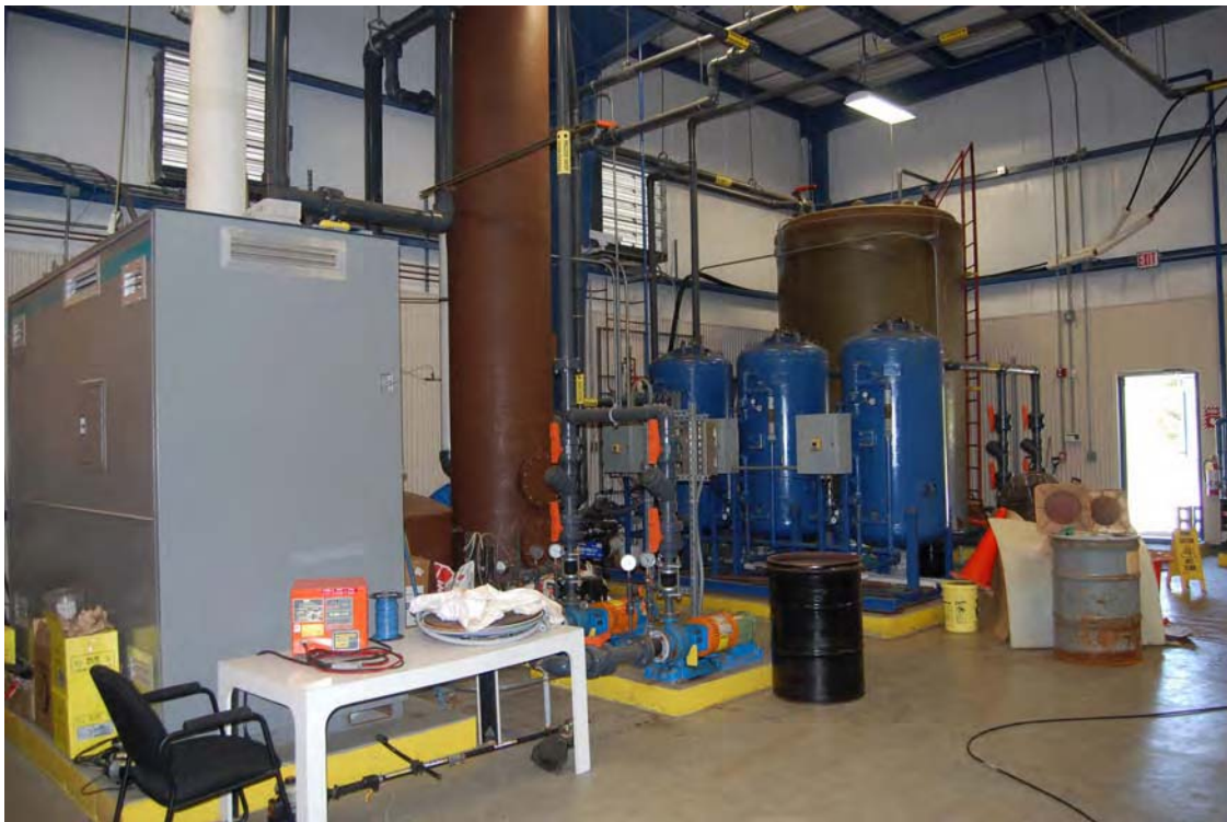
Photo Number: 10 - Air-stripper, multi-media filters, backwash tank. Date: May 29, 2008
