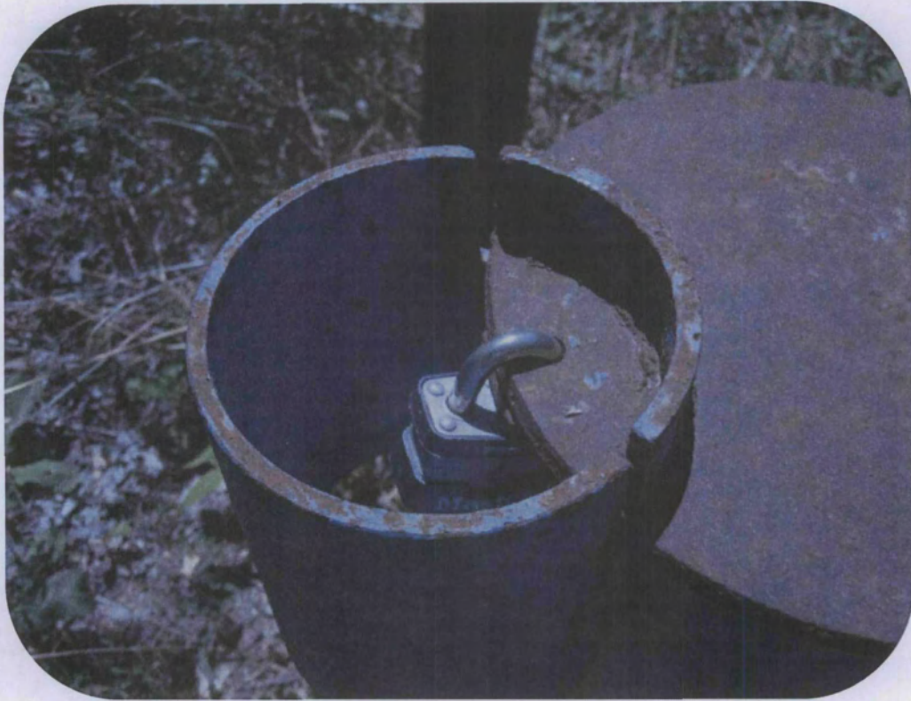
Photo 13: Lock with guard on MW 6M.
