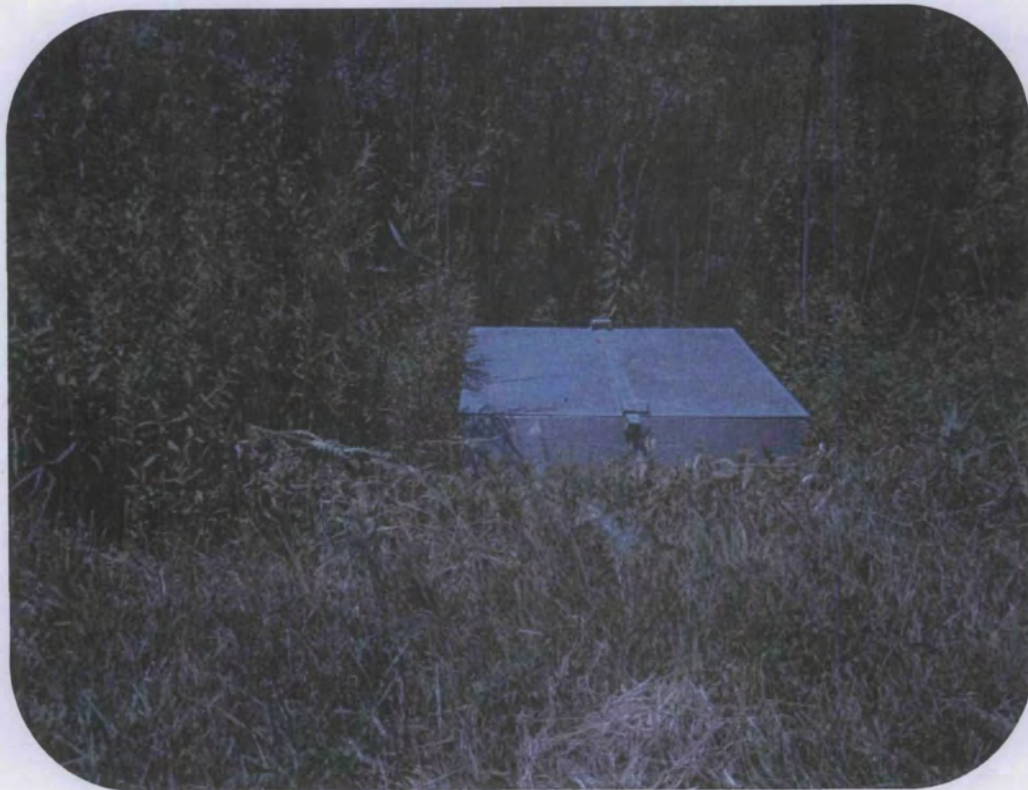
Photo 9: Condensate sump along western edge of fence.
