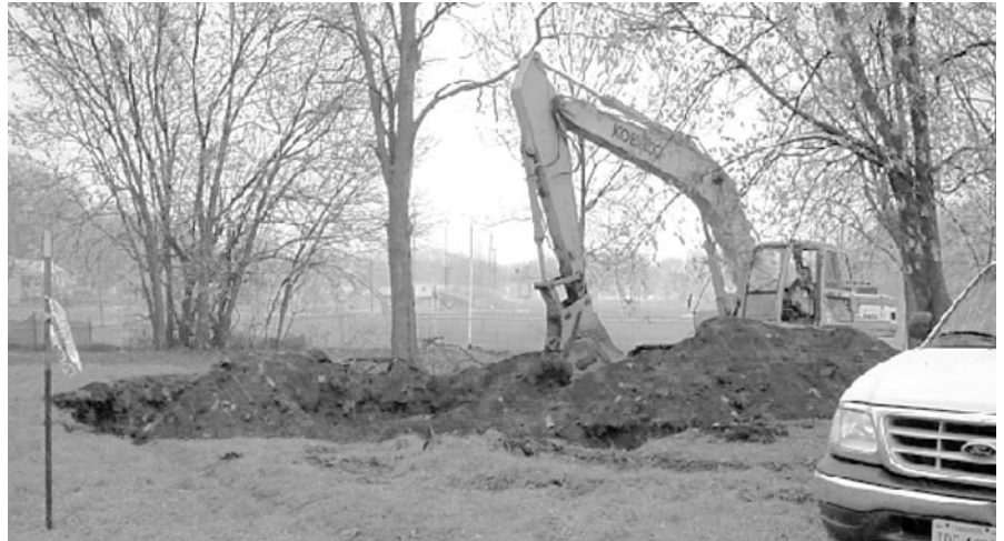
EPA excavates lead-contaminated soil at the NPL-1 area.
