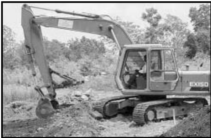
Soil is excavated at NPL-8 to initiate the treatability study.
