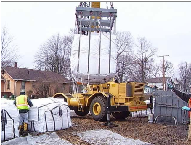
Contractors load contaminated soil into specially designed bags for removal.
