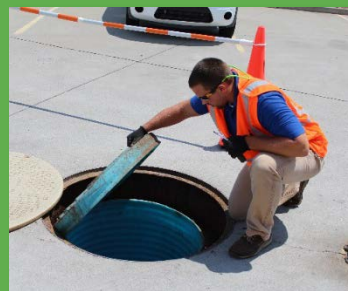
Inspecting a containment sump
