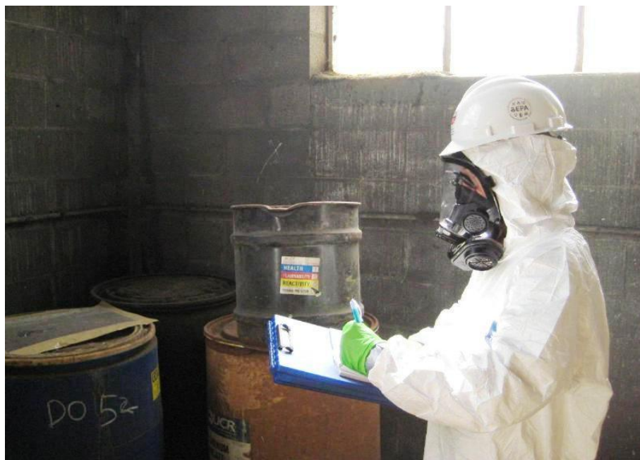
An EPA emergency responder checks out some of the numerous drums containing dangerous acids and flammable liquids discovered in the abandoned Advance Plating facility. The drums will be removed and the site secured during the cleanup project that is expected to last until March.
