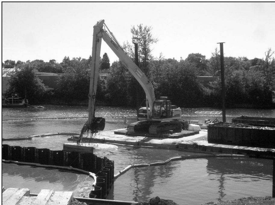
PAH-contaminated sediment is dredged from the Sheboygan River during the 2011 emergency cleanup.
