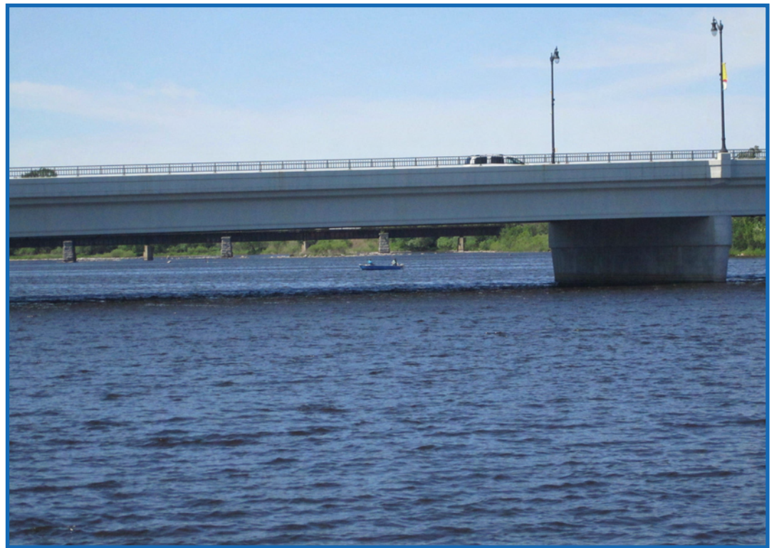
Bridge Street bridge over the Menominee River
