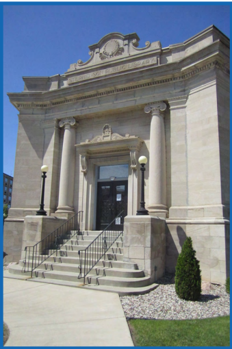
Entrance of Stephenson Public Library, original building.
