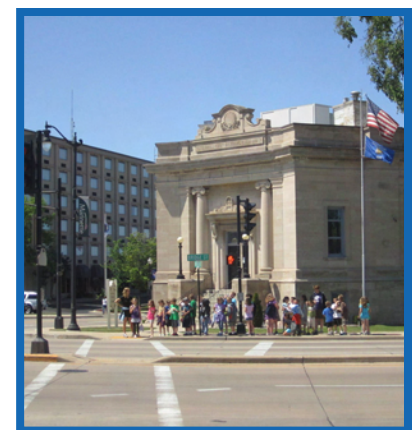
Entrance of Stephenson Public Library, original building.
