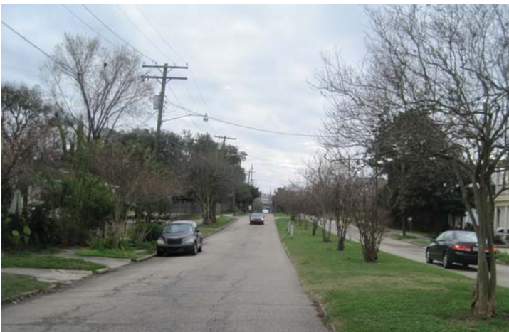
Figure 29: This image shows the current condition of East Boulevard.
