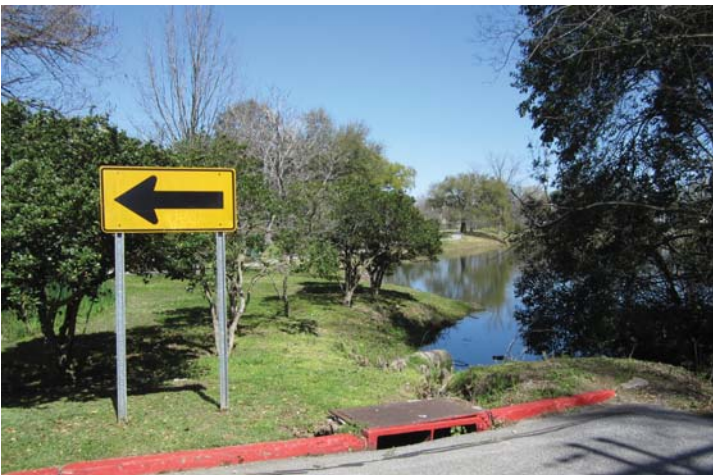
Figure 47: This photo shows the existing conditions where North 7 th Street ends at Arsenal Park.
