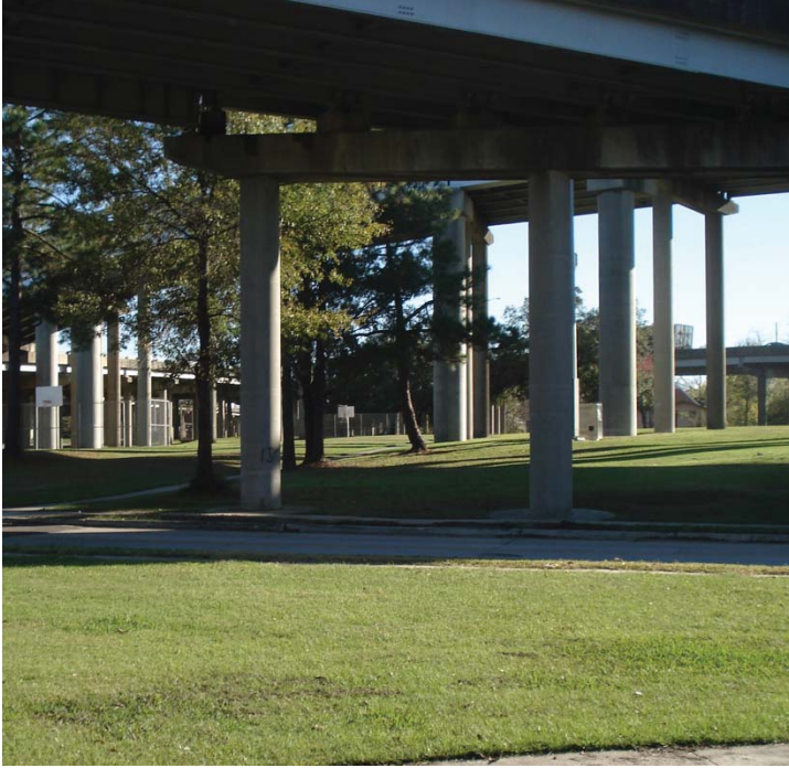
Figure 8 Interstate structures dominate most of the park, with some open space between the supports.
