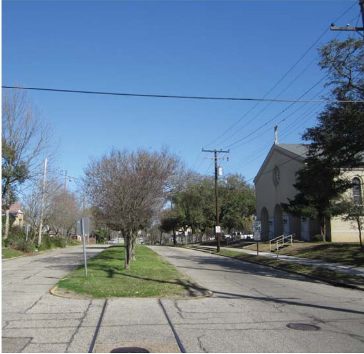
Figure 11 Looking north on East Boulevard, the old streetcar tracks are still evident. The trees planted in the median do not appear to be maturing, likely because the rail bed was not removed before the trees were planted.
