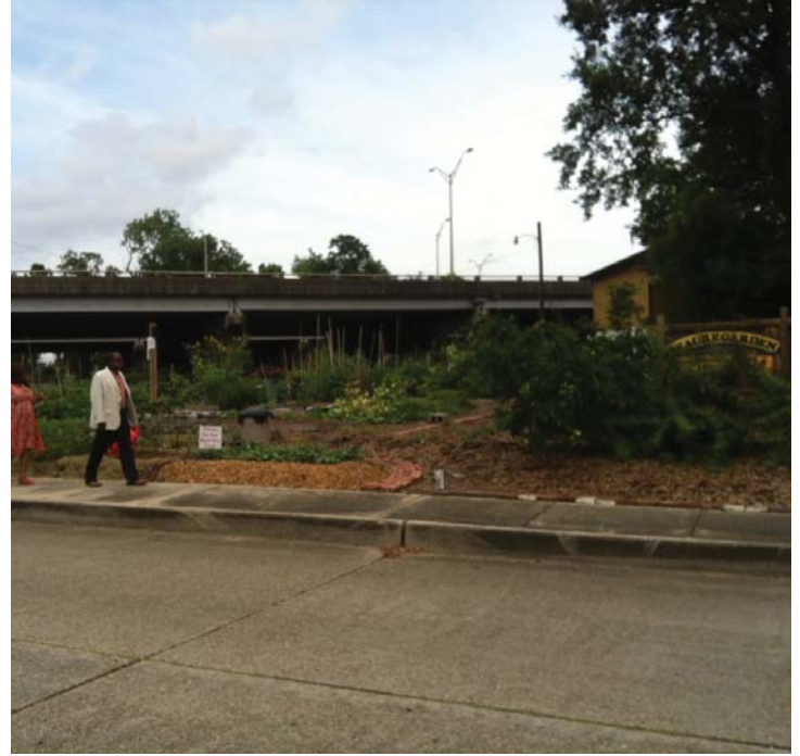
Figure 12 From Louisiana Avenue looking east, The greenway would continue under the interstate.
