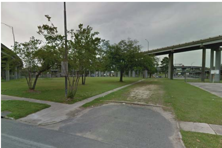
Figure 24: A view of Expressway Park's current condition.
