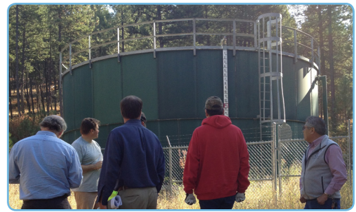
Figure 12. System Inspection for Mapping
