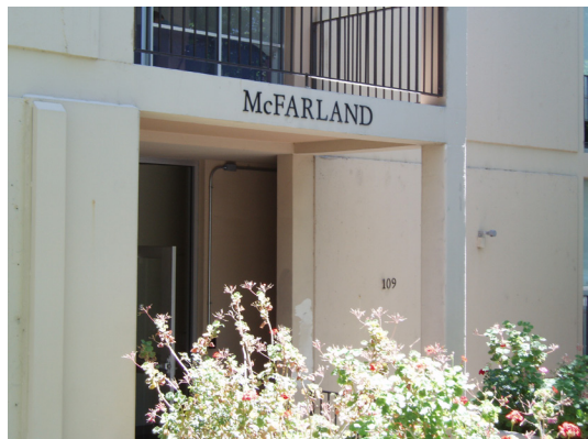
McFarland midrise will be fully sprinklered by the end of summer 2013
