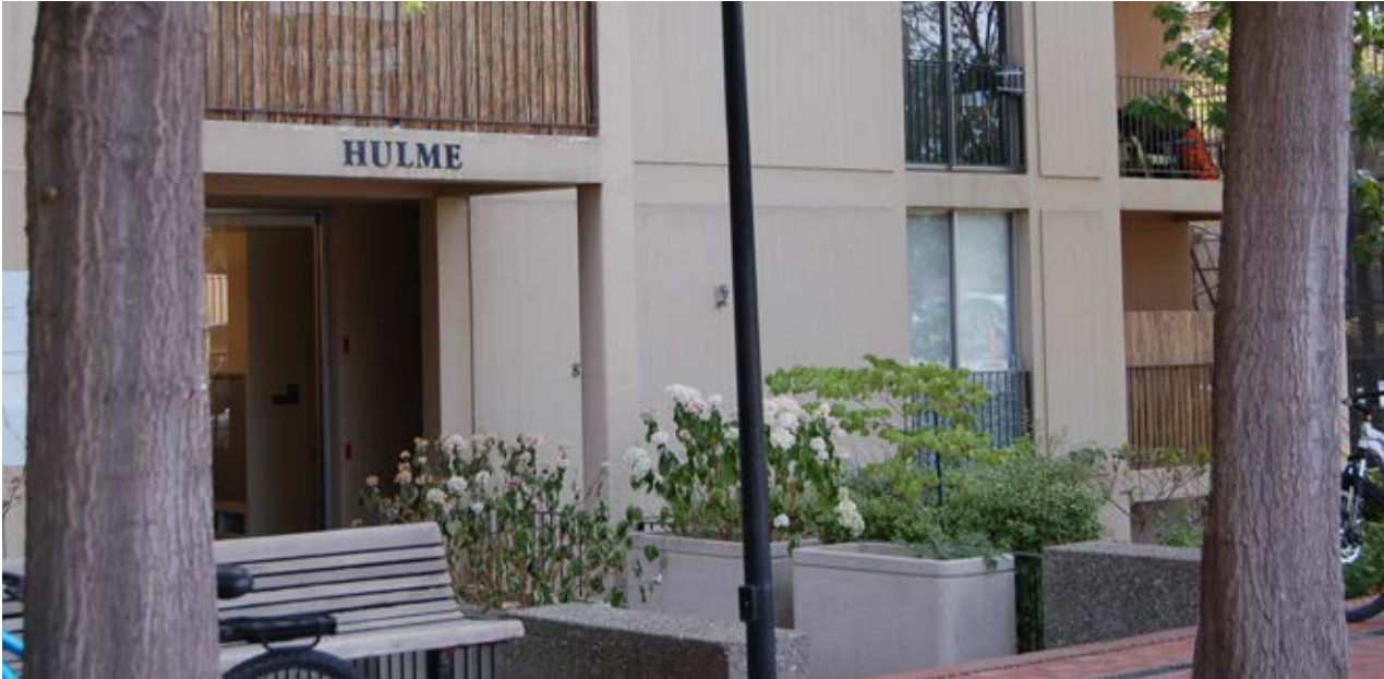
A fire sprinkler system retrofit in the Hulme Midrise will be fully installed by the end of the summer, 2014.
