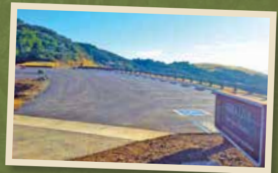
BALD MOUNTAIN PARKING: Funded by a grant from the Coastal Conservancy, the new parking area and restroom provides visitors an access point for the future trail to the Mount Umunhum summit.
